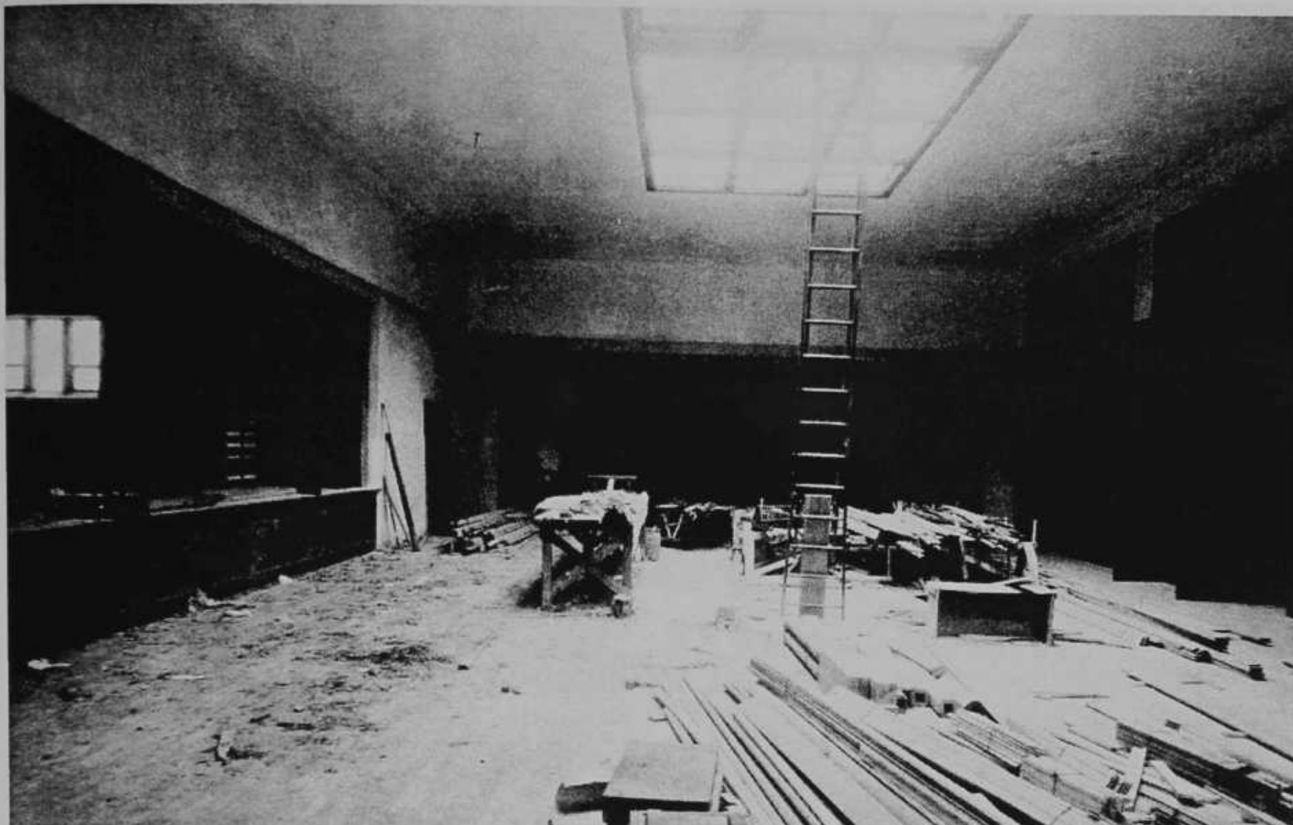
Gymnasium under construction
