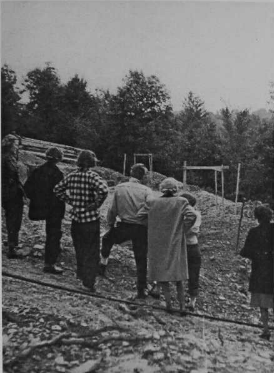
Beginning construction of original lodge at Akita - 1948
