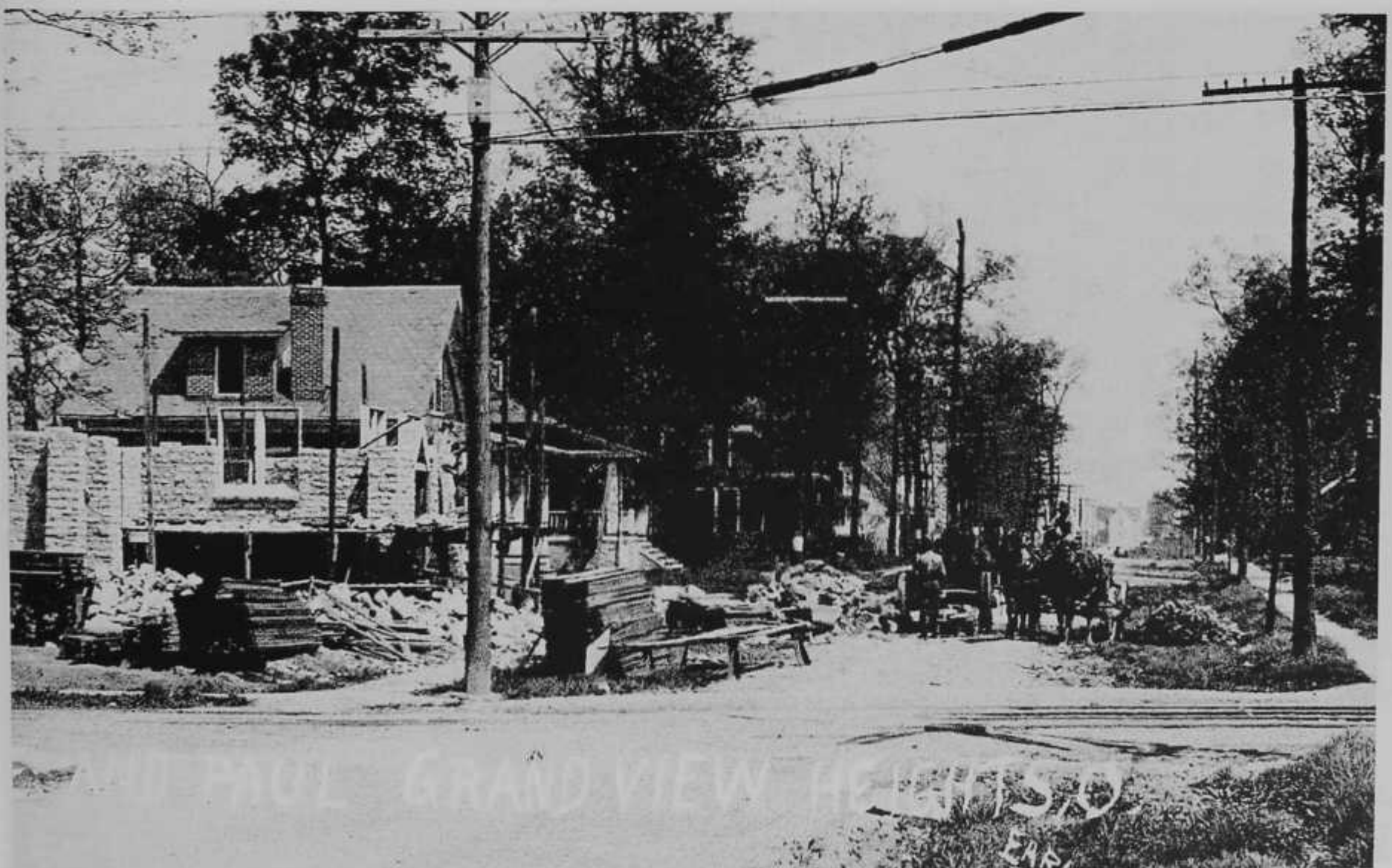
Construction of Grandview Heights Congregational Church. Note horse-drawn wagon carrying stone. (Photo courtesy of Grandview Heights Marble Cliff Historical Society.)
